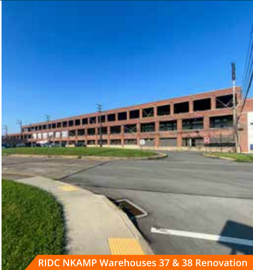
RIDC NKAMP Warehouses 37 & 38 Renovation
