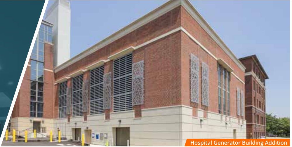
Hospital Generator Building Addition
