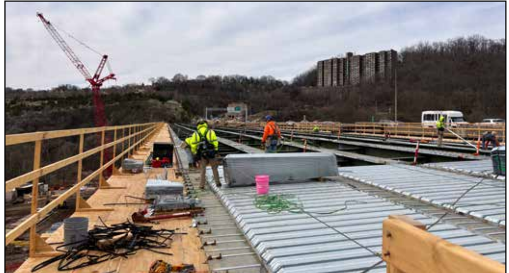
On the cover: Ongoing PennDOT work on the "sliding bridge" upgrade outside the Squirrel Hill tunnel. Image courtesy of PennDOT.
