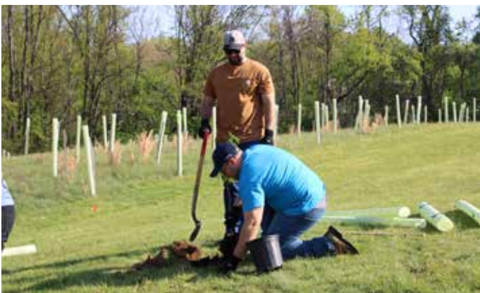
Armand Dellovade of Mohawk Construction checking the work of Zane McShane of Brayman Construction.
