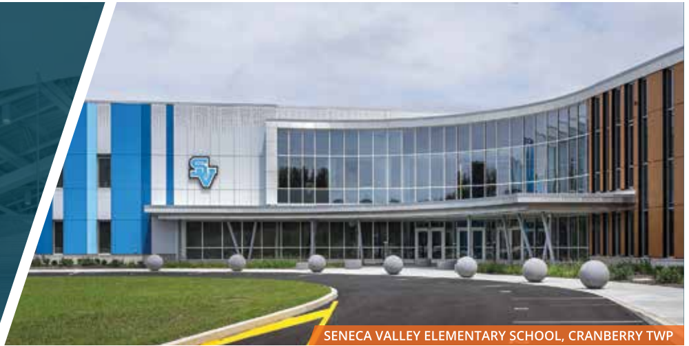
SENECA VALLEY ELEMENTARY SCHOOL, CRANBERRY TWP
