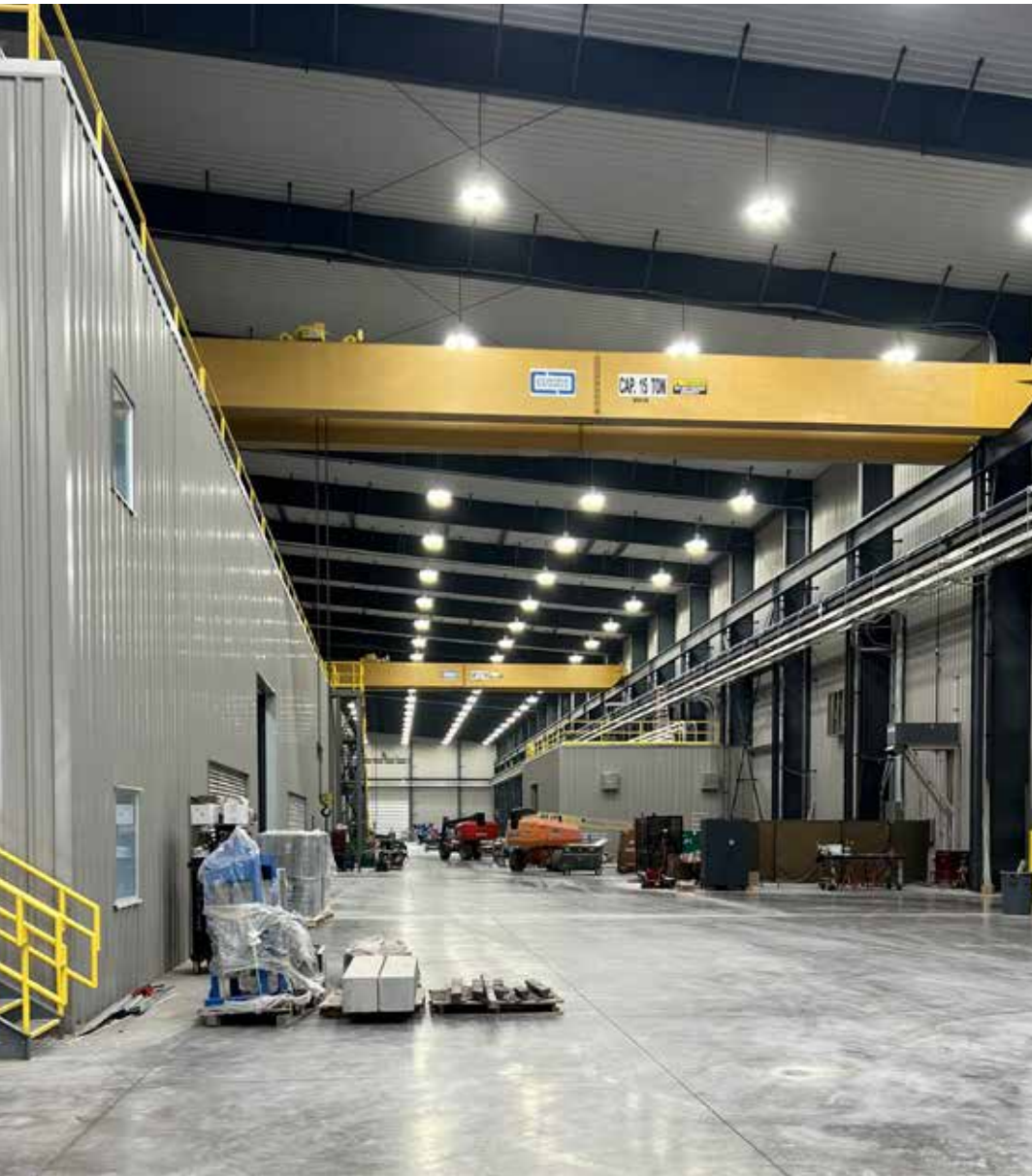
Foundations for the manufacturing equipment required major changes to the building foundations as construction was underway. Photo by Stevens Engineers and Constructors.
