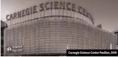
Carnegie Science Center Pavilion, 2018
