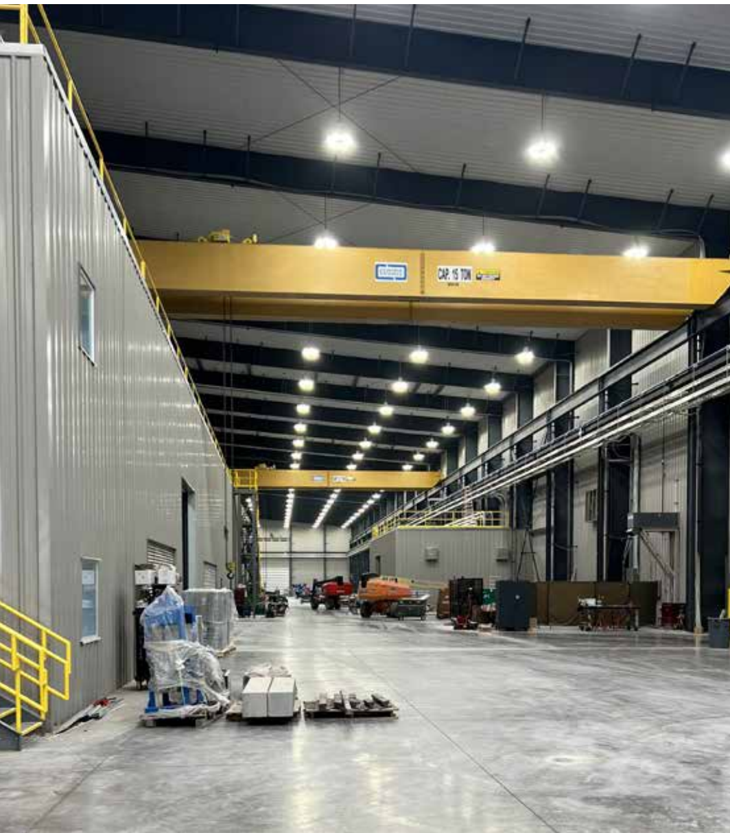
Foundations for the manufacturing equipment required major changes to the building foundations as construction was underway. Photo by Stevens Engineers and Constructors.
