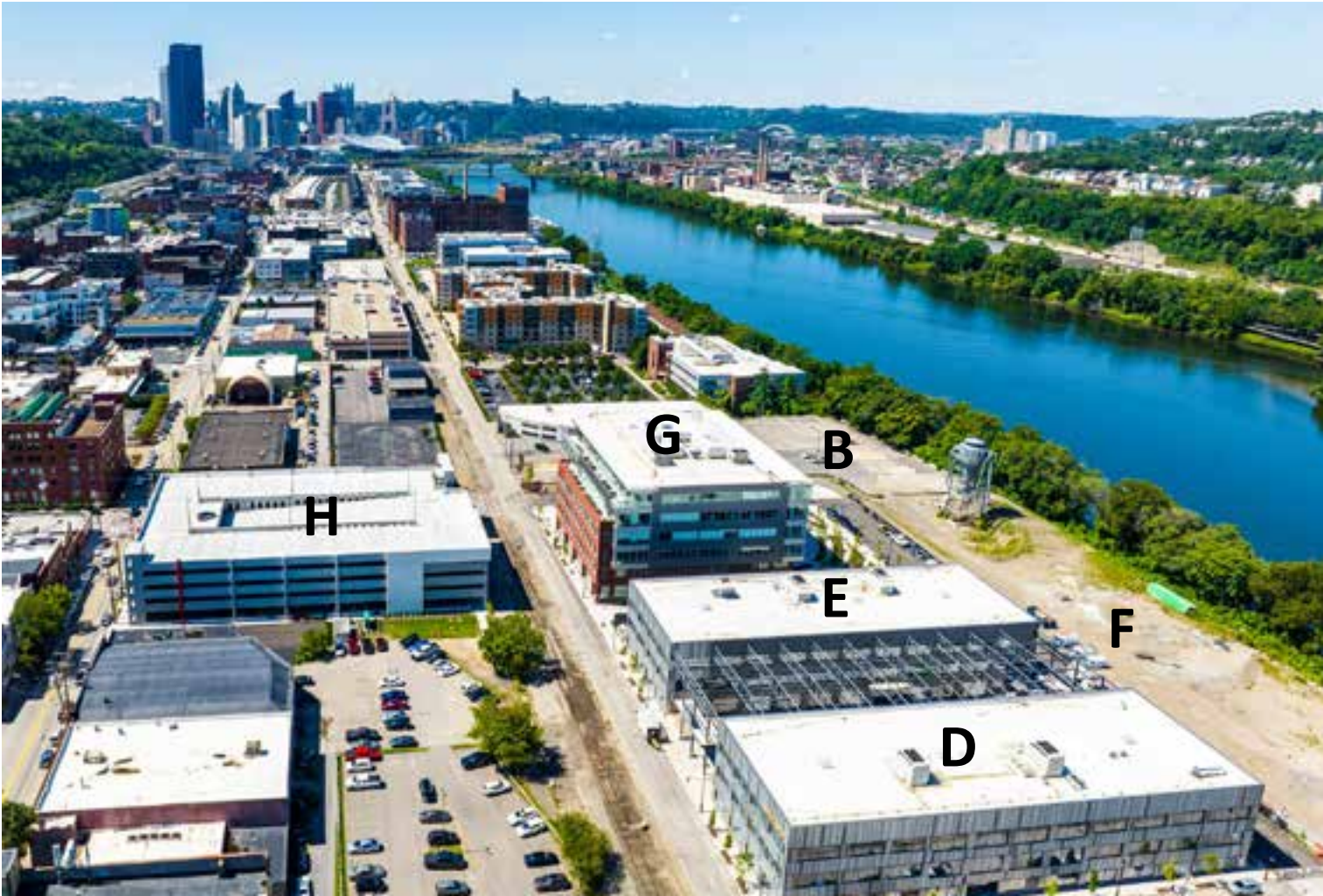
Construction has been completed on The Hive (H), The Stacks (E and D), and 75 Hopper Place (G) in the second phase of 3 Crossings. The proposed office buildings (B and F) totaling 300,000 square feet have been stalled by the disruptions in the office market and commercial real estate financing. Photo courtesy Oxford Development Co.
