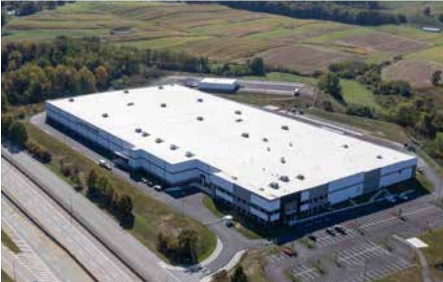
New warehouse for Frank B. Fuhrer Wholesale in Salem Township was completed by ARCO Pittsburgh in fall 2023. Photo by Dronegenuity.
