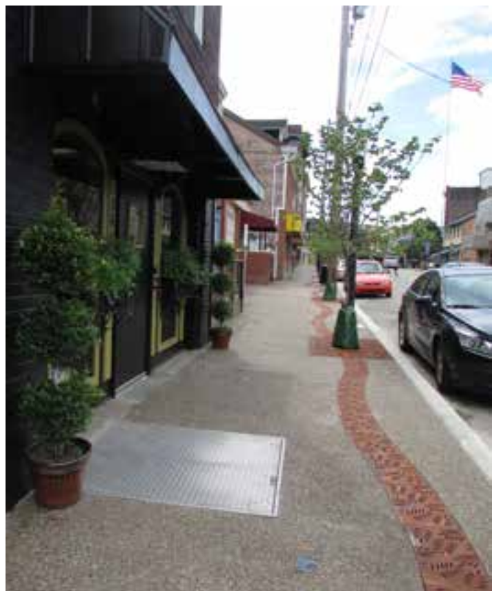
One of the stormwater mitigation strategies employed in Etna involves a connected series of drains set in a winding pattern in the sidewalks. Photo courtesy Borough of Etna.
