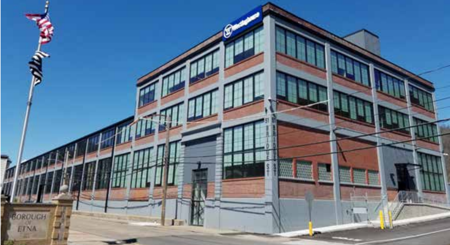
51 Bridge Street sits at the entrance to Etna's business district.
