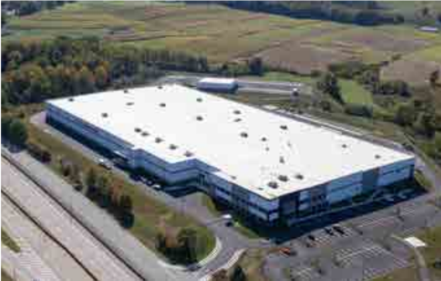
New warehouse for Frank B. Fuhrer Wholesale in Salem Township was completed by ARCO Pittsburgh in fall 2023. Photo by Dronegenuity.
