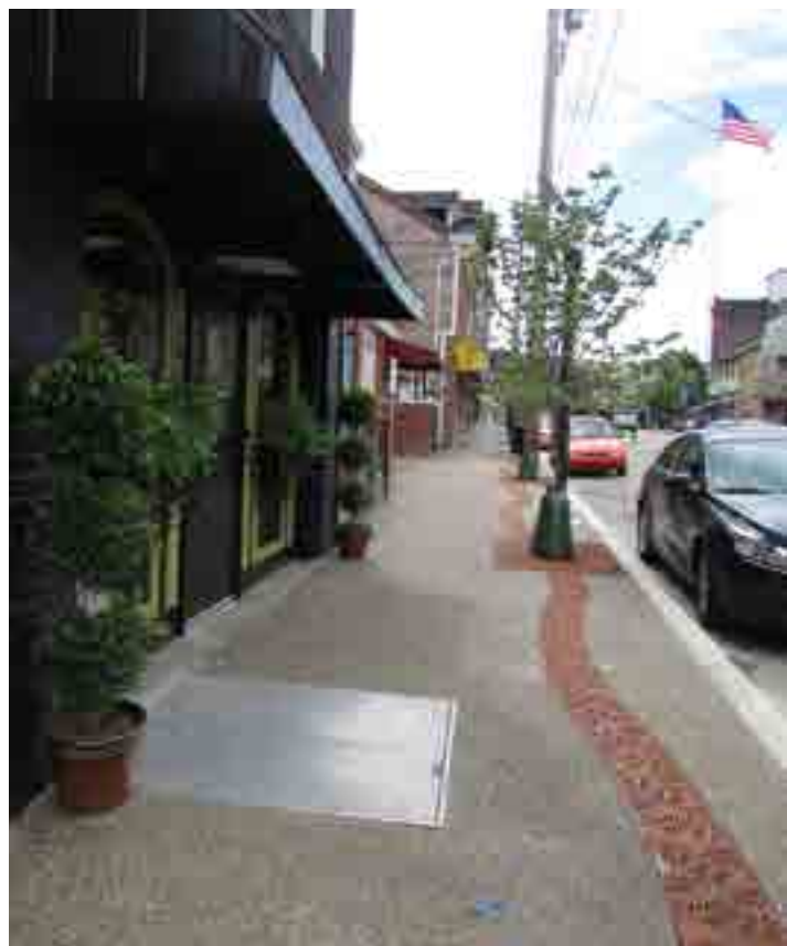
One of the stormwater mitigation strategies employed in Etna involves a connected series of drains set in a winding pattern in the sidewalks. Photo courtesy Borough of Etna.
